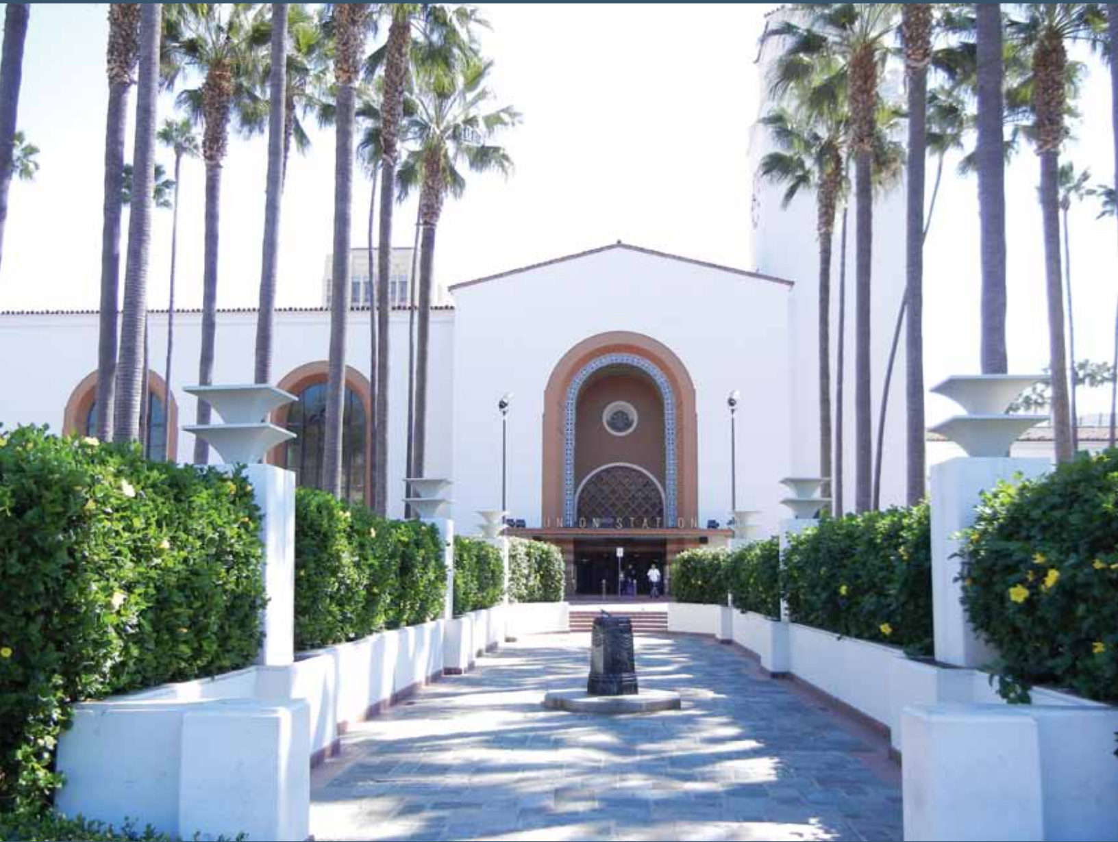
Union Station, Los Angeles
